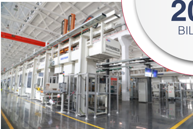
Finish Machining Line for National VI compliant Engine YCS04/ YCS06 cylinder block machining.
