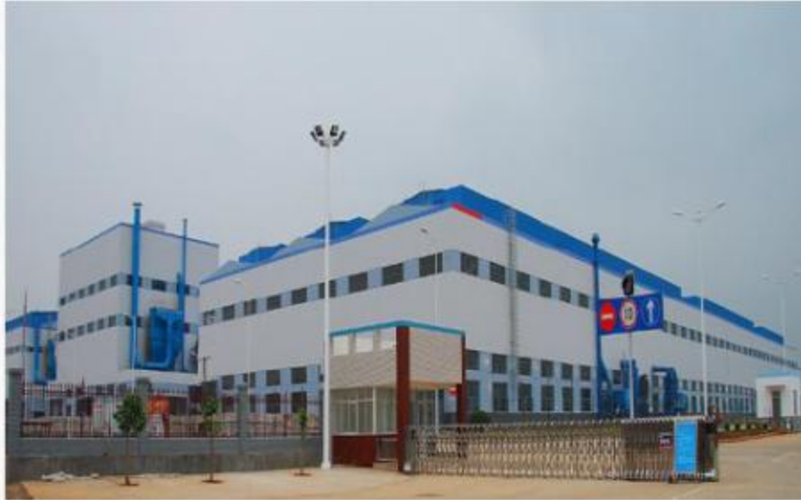
New Foundry Phase 1
